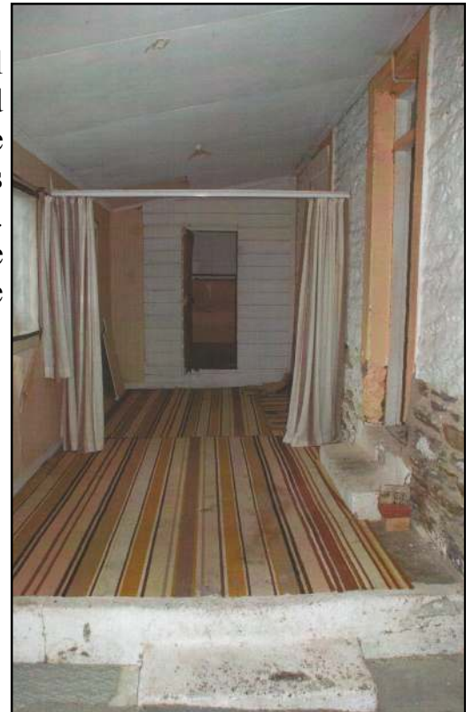
Interior Before Renovation: This photo taken from the floor level of the older cottage shows the four steps up to the level of the second cottage. The wall on the right still has its original whitewash of lime, mutton fat and cream.
