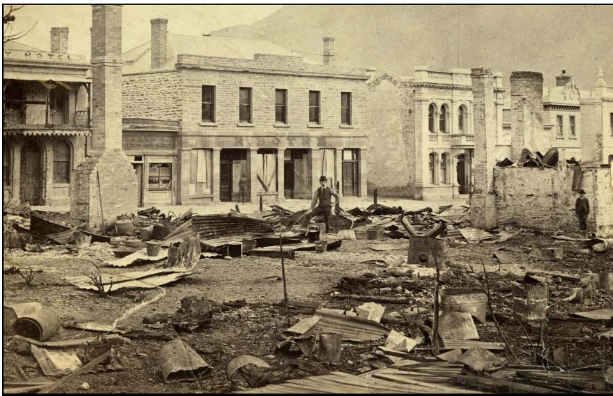
Ballarat Street after the fire
