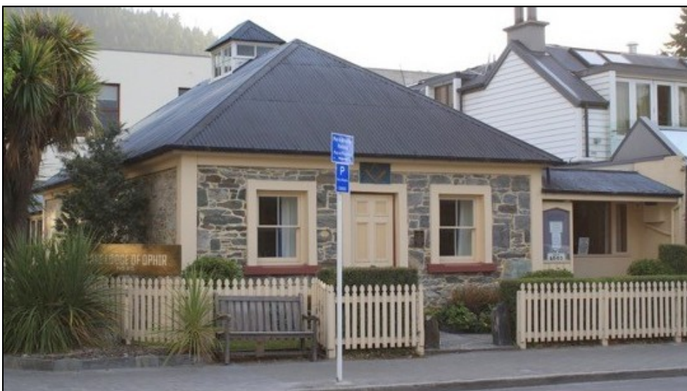
After the restoration project in 2008
